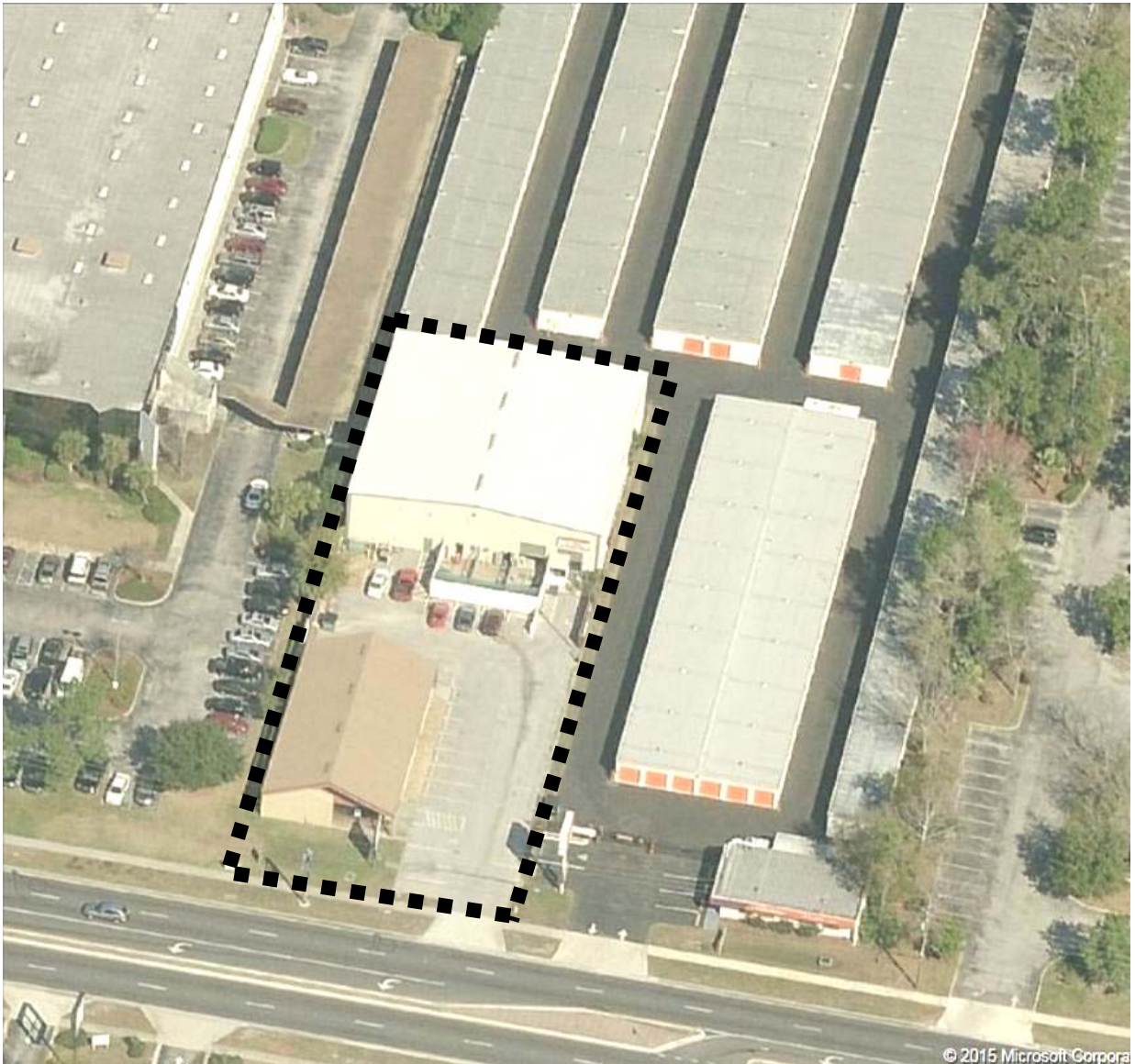
Aerial view of site. Camp bow Wow is large white building at the rear of the property.
